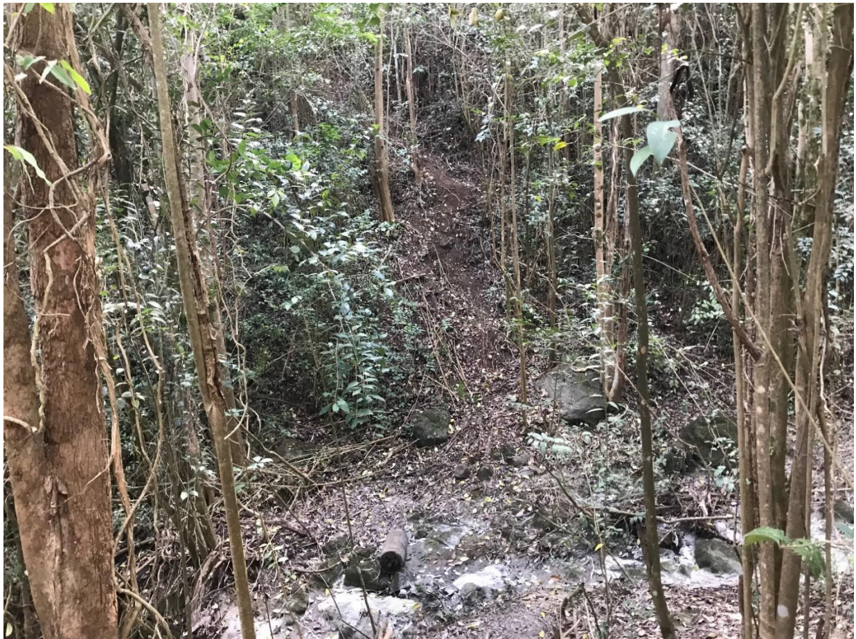
Photo Point 04 – MZ 4 – Base of unstable mound to be removed – Privet habitat along corridor
