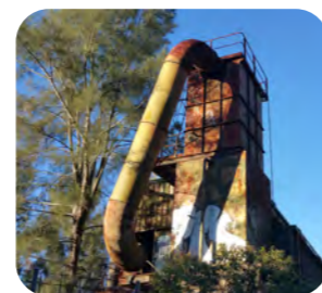
Adaptive reuse of the Crusher Plant
