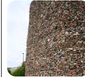
Sandstone Welded Mesh Gabion Wall
