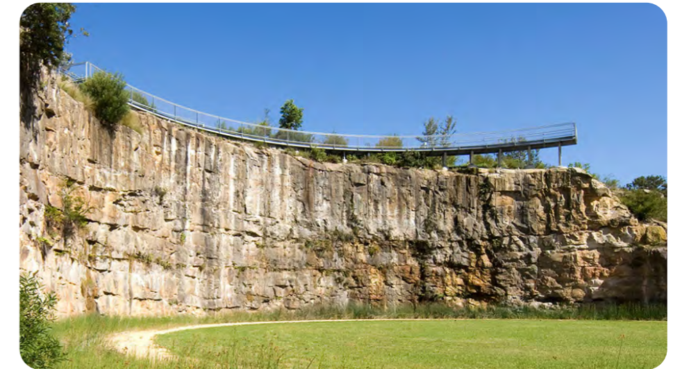
BP Site, Waverton (North Sydney Council) The rough quarry faces of this former oil storage site contrast with the simple curved geometry of the steel viewing walkway.
