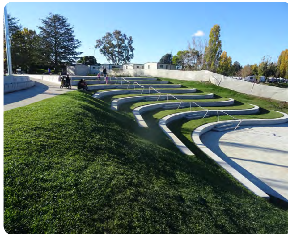
Queanbeyan Riverfront (CLOUSTON Associates) The level changes between street front and river provide opportunities for seating and performance spaces at the water's edge.
