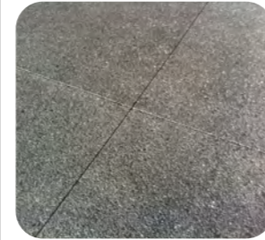
Exposed Aggregate Concrete (Feature Paving)
