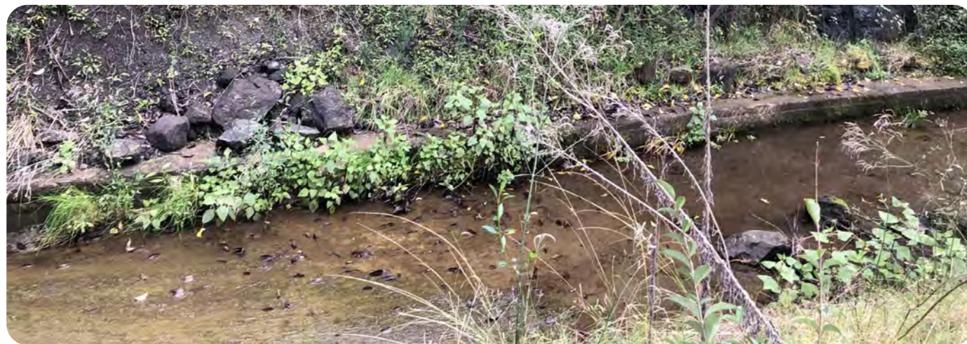
Concrete drainage channel
