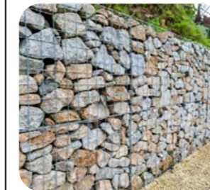
Breccia Welded Mesh Gabion Wall
