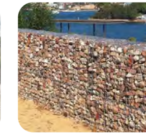
Low Welded Mesh Gabion Wall
