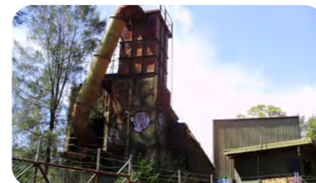
Photo 4: The Crusher Plant
