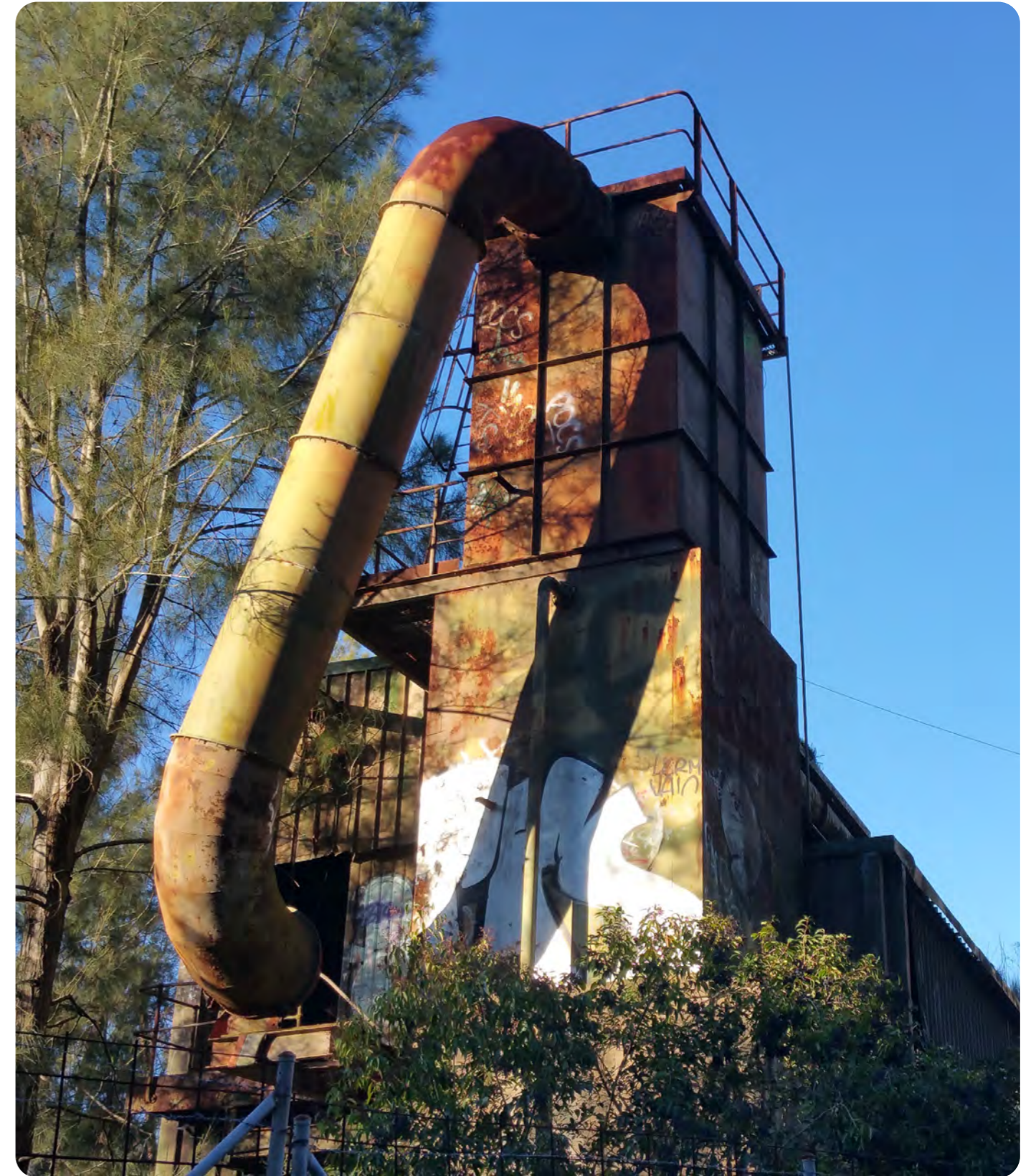
Crusher Plant tower
