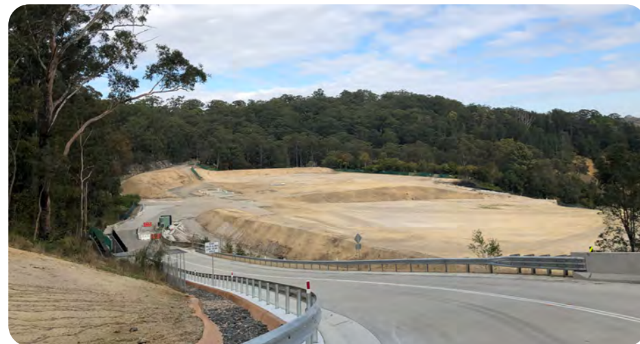
Existing road from Bridge Road to OMV
