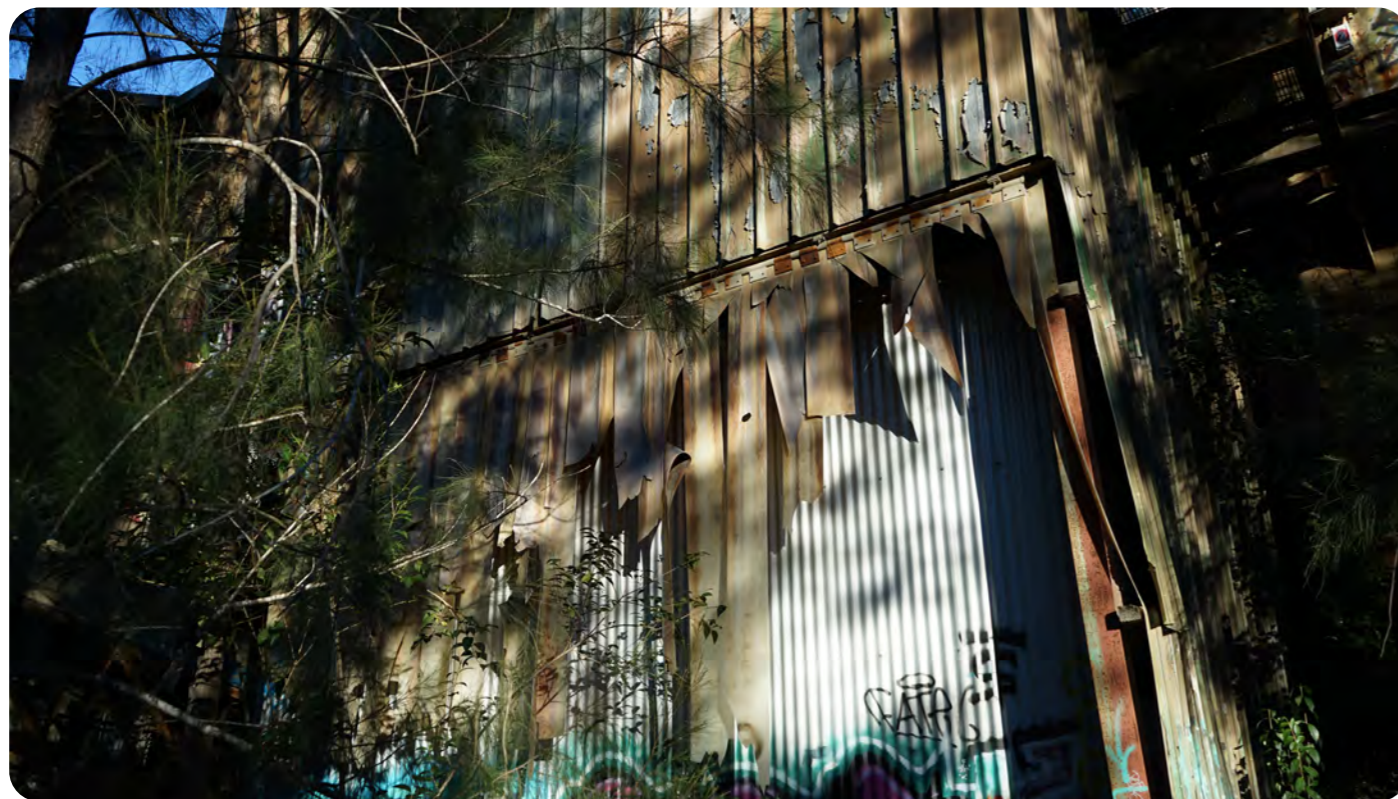
Crusher Plant tower base
