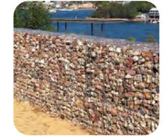
Low Welded Mesh Gabion Wall
