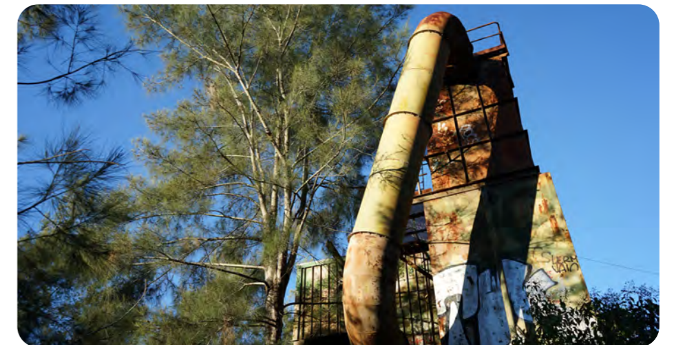
Existing Crusher Plant
