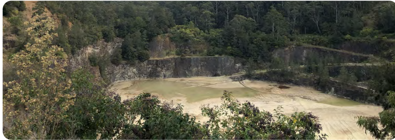
Hornsby Quarry Walls
