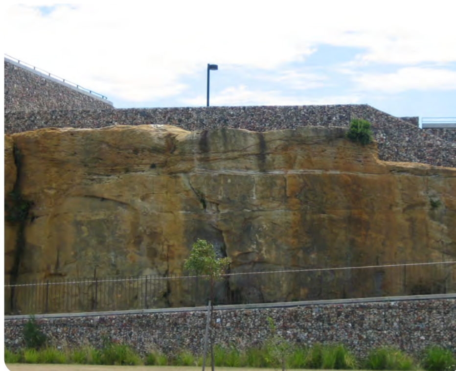
Ballast Point Park (McGregor Coxall) Layering of existing industrial modified landform and new parkland elements to create a park which celebrates the history of the site while providing a green park for passive recreation.
