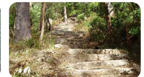
Photo 6: The Heritage steps have been restored.
