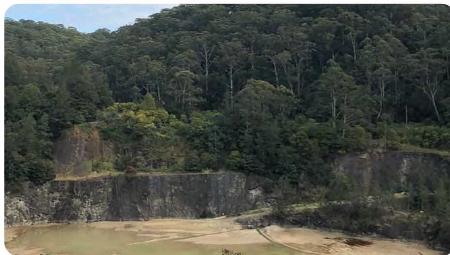
Existing Quarry north west corner - cantilever path to provide DDA access into void
