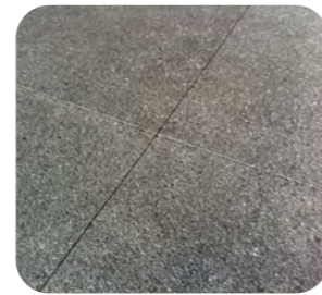
Exposed Aggregate Concrete
