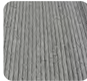
Raked Concrete Footpath
