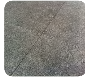
Exposed Aggregate Concrete
