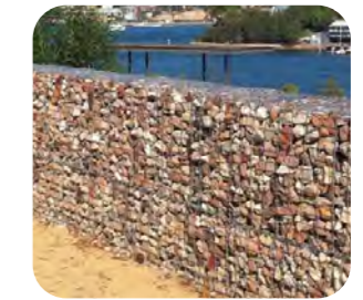
Low Welded Mesh Gabion Wall
