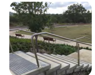
Stainless Steel Handrail Wall
