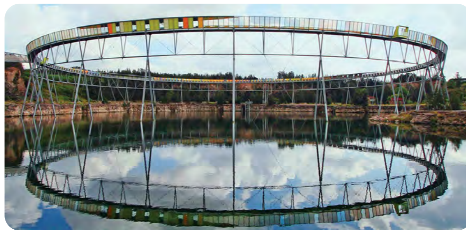
Floating ramps and walkways
