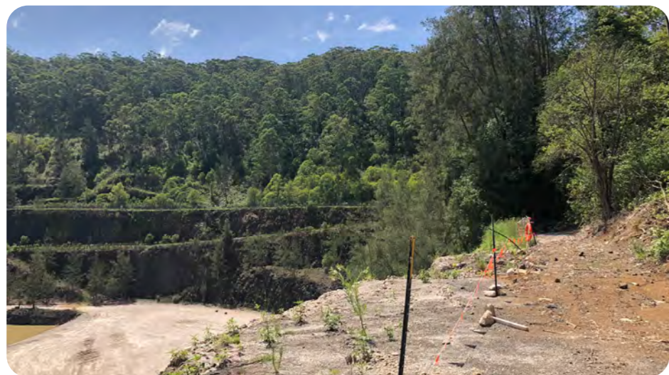
Existing Quarry RL88 bench - cantilever path and stairs to provide access
