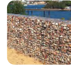
Low Welded Mesh Gabion Wall
