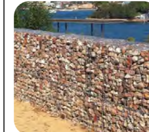
Low Welded Mesh Gabion Wall
