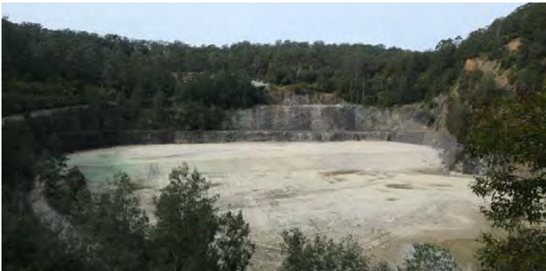
Figure 1 – View from the western side of the now abandoned Hornsby Quarry looking east towards Old Mans Valley. (Photo: Arterra 25 July 2019)
