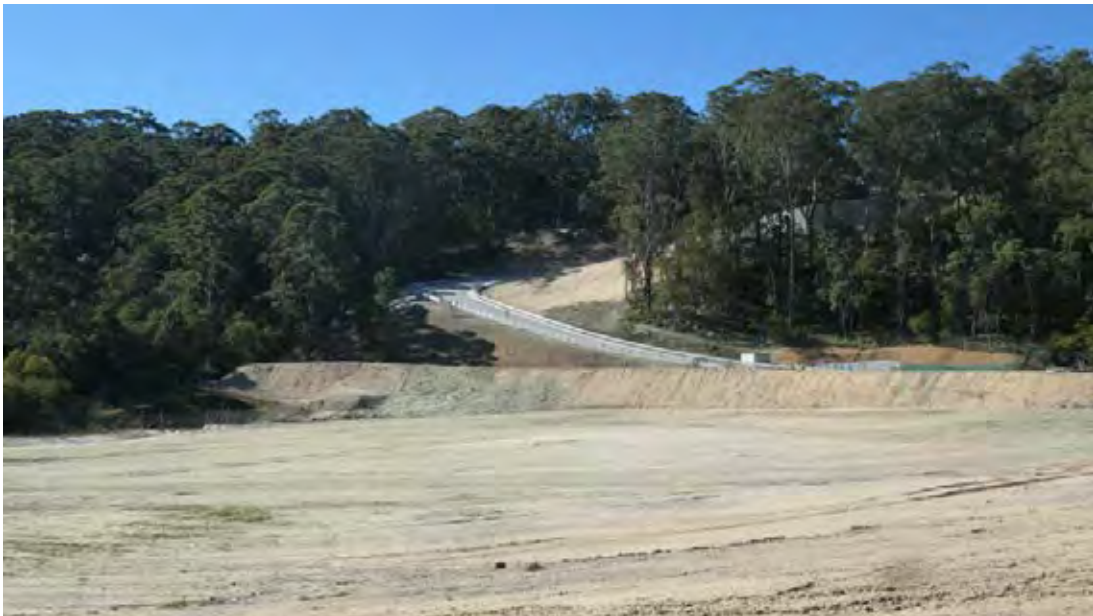
Figure 7 – View of the northern end of the Old Man’s Valley fill area and the newly constructed driveway leading to Bridge Road. (Photo: Arterra 22 July 2019)
