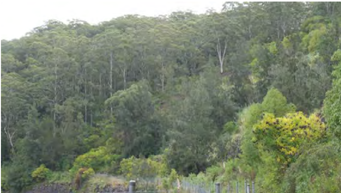
Figure 9 – Northern fill slopes - at right and view to western edge of the fill slope and its interface with the more natural vegetation of the Blue Gum and Blackbutt Gully Forest beyond. (Photo: Arterra 25/7/19)
